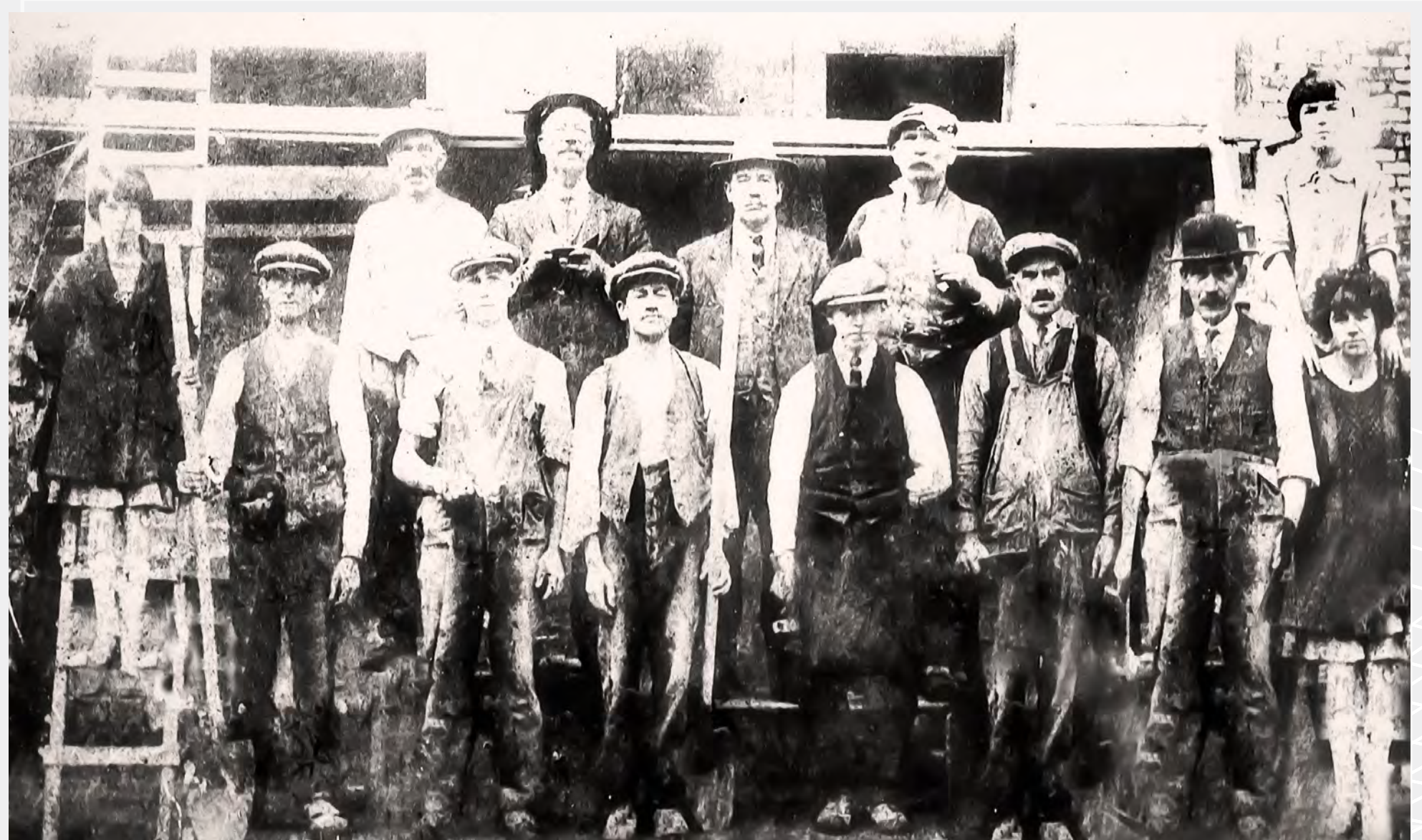
Patrick Elliott (4th from left) with the original construction team
